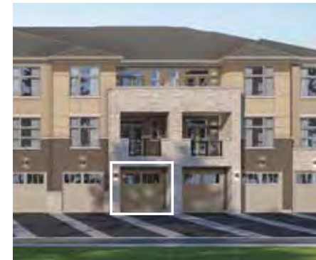
REAR, Interior Unit
