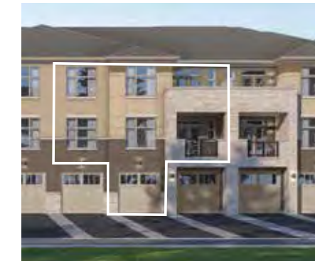
REAR, Interior Unit
