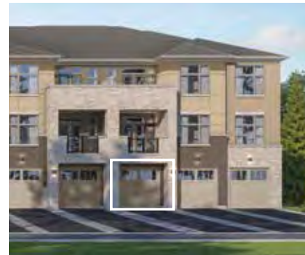
REAR, Interior Unit
